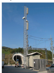
Stazione radio base (BTS) Base Transceiver Stations (BTS)
