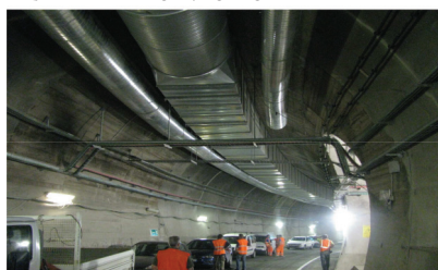
Controllo fumi in finestra Smoke control system in the escape tunnel
